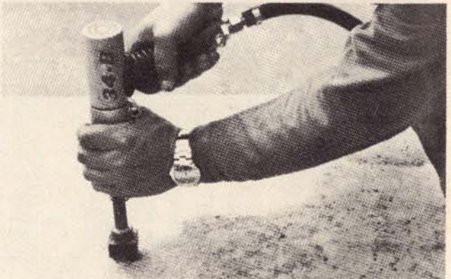
On the construction site: Cleaning, stripping, roughening.
